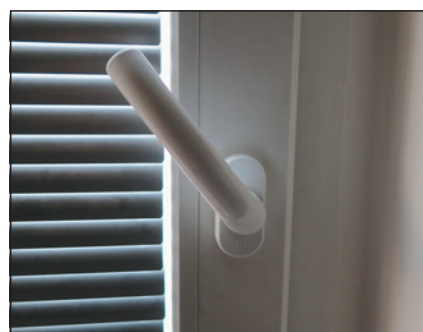
▲ Obr. 4 ● Mikroventilace 4 mm
