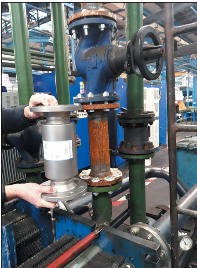
▲ Obr. 6 ● Draka Kabely Prysmian Group 1
